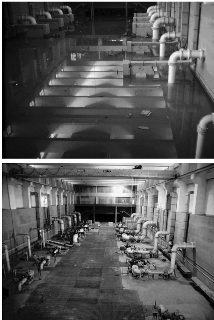
FIGURE 12.30 Kuwaiti Central Water Pumping Station before and after Repairs
