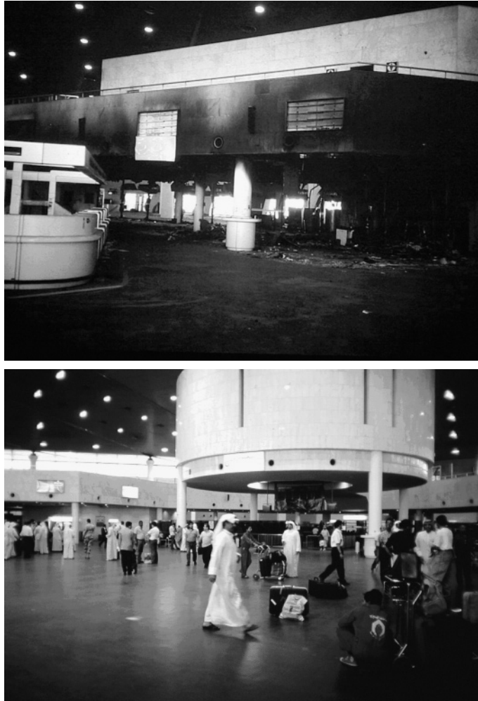
FIGURE 12.20 Airport Lobby Restored in 30 Days with “Task Order” Contract
