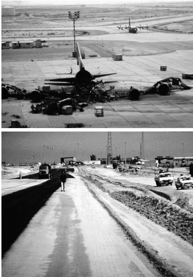
FIGURE 12.18 Project managers made transportation system repairs a top priority
