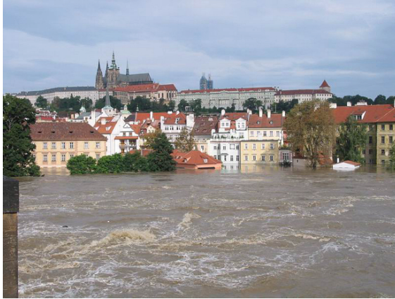
Figure 2. Floods in Prague 2002
