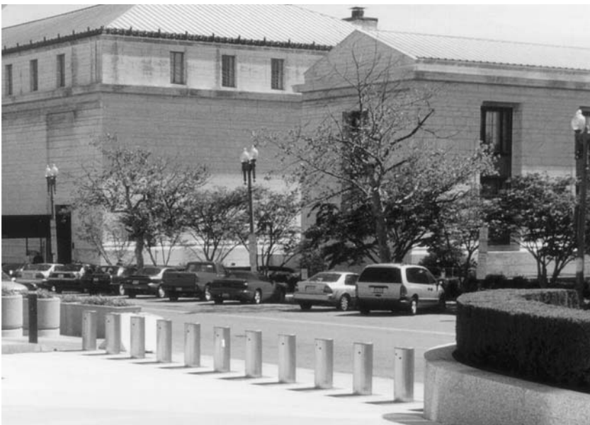
FIGURE 9.4 Raised stainless steel bollards protect access to the U.S. Department of State headquarters. (Courtesy of Delta Scientific, Inc.)
