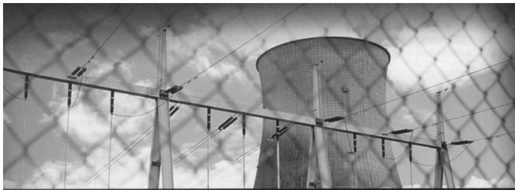
FIGURE 1.2 A nuclear power facility.
