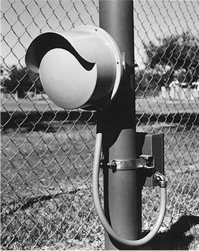
FIGURE 9.6 Capacitive field effect. (Courtesy of Southwest Microwave, Inc.)
