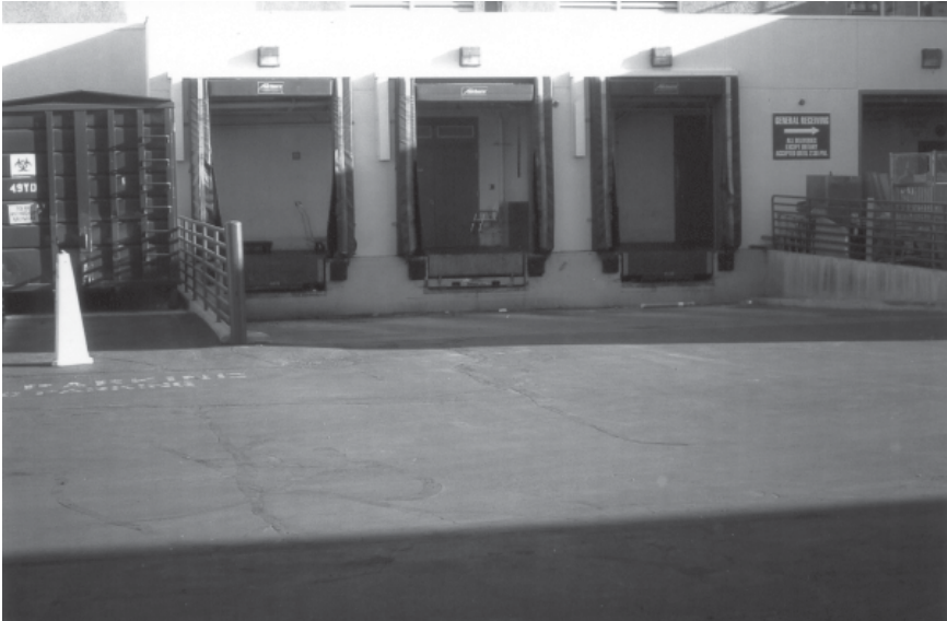
Figure 5-6. Loading dock with roll-up doors. (Photo by Robert Reid, 2004)
