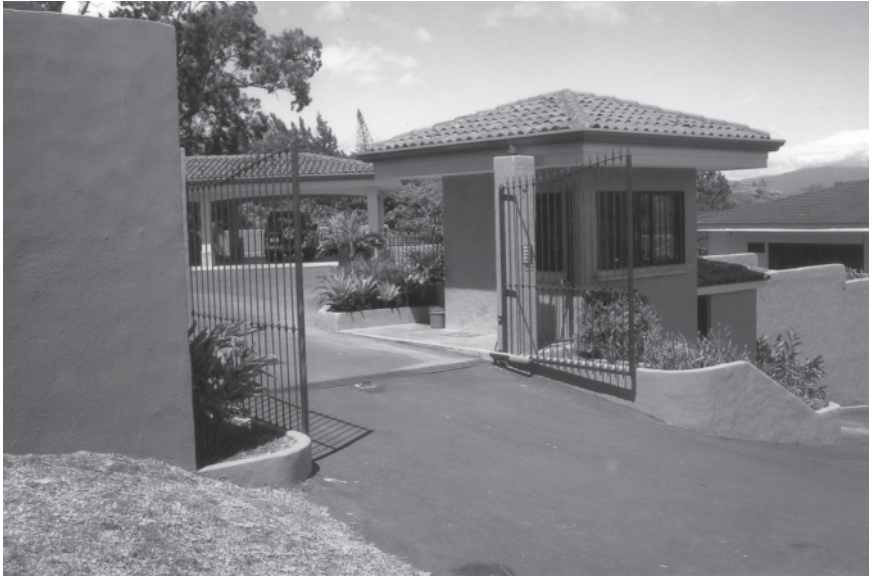
Figure 3-15. Guard house for an apartment complex. (Photo by Robert Reid, 2004)
