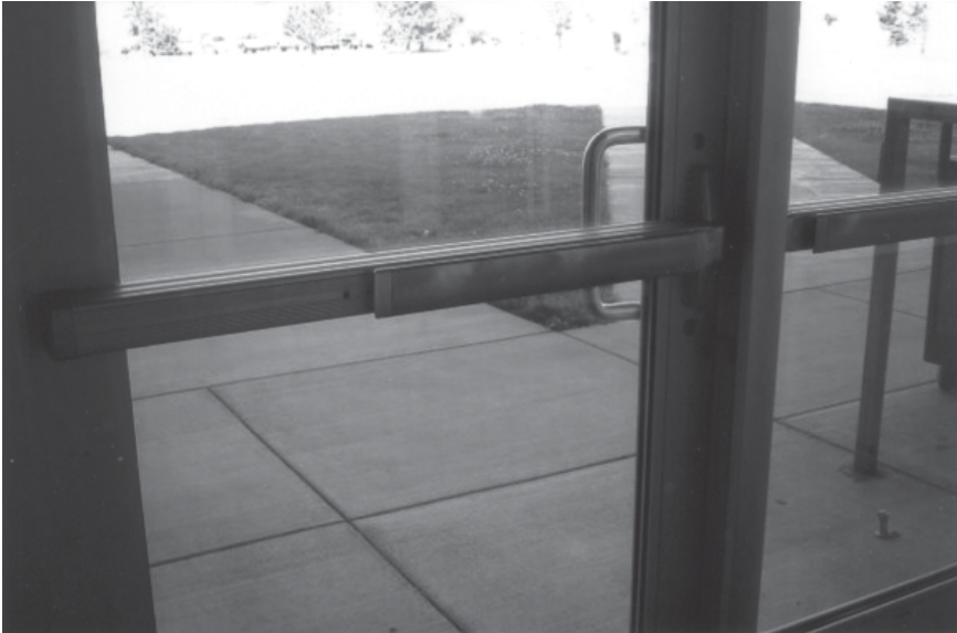
Figure 6-6. Panic Hardware. This figure shows door hardware called “Panic hardware.” The bar across the door will release the door. These bars are required in locations where there are large groups of people like schools or auditoriums. ( Photo by Robert Reid, 2004 )
