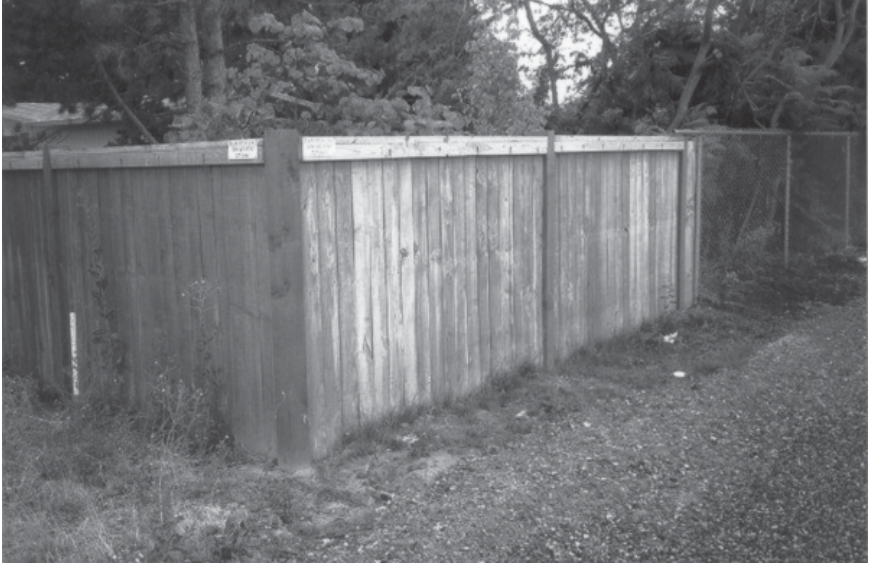
Figure 3-8. A typical wood fence. These fences do not provide a great deal of security, but they do obstruct vision, preventing intruders from knowing location of material or equipment inside the area. (Photo by Robert Reid, 2004)
