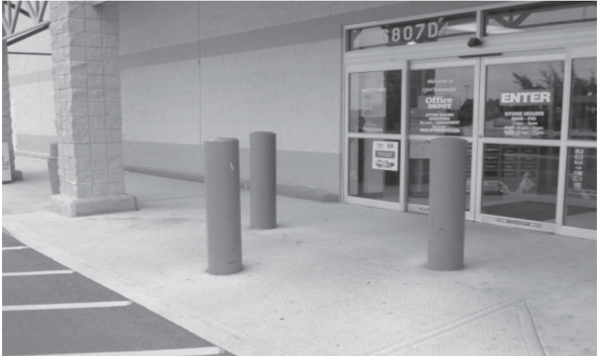
Figure 3-3. Pipe Bollards protect entrances to facilities by vehicles. (Photo by Robert Reid, 2004)
