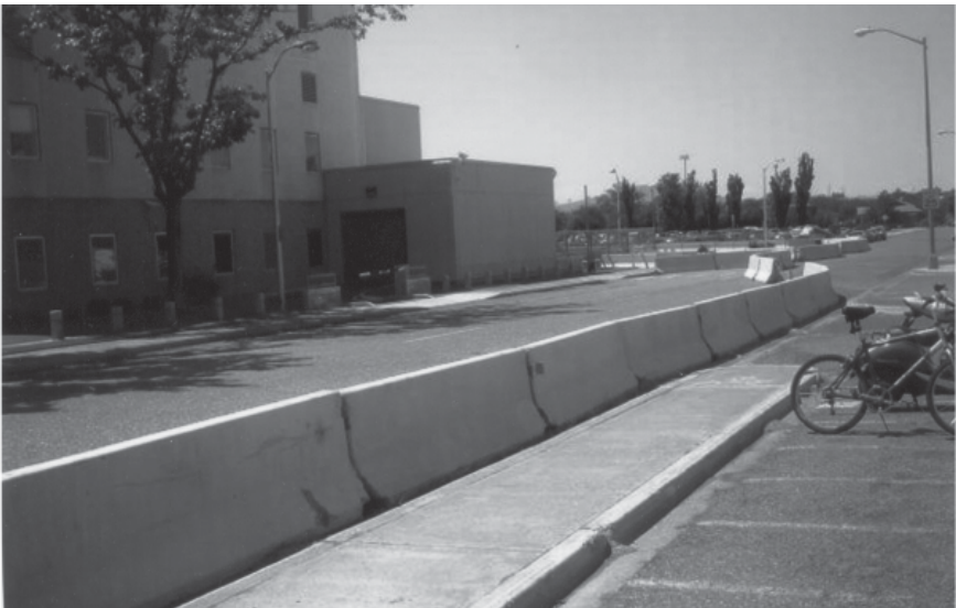
Figure 3-2. A jersey barrier is a good temporary security measure to control traffic flow. (Photo by Robert Reid, 2004)
