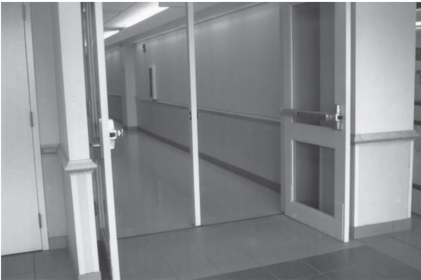
Figure 5-4. Double door. Photo by Robert Reid, 2004.
