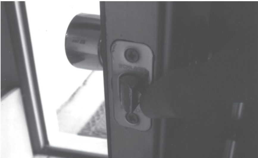
Figure 6-2. Latch and Dead Latch. The latch is the portion of the door hardware that catches in the strike pocket and holds the door closed. A “dead” latch is that part of the latch that locks the latch in place. The dead latch is forced back by the strike pocket. (Photo by Robert Reid, 2004)
