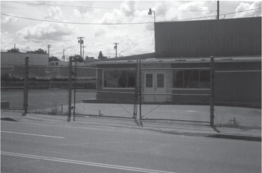
Figure 3-11. A typical chain link double hinged gate. (Photo by Robert Reid, 2004)
