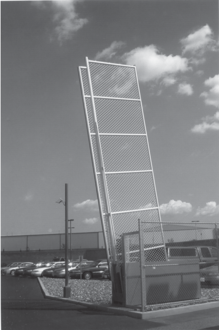
Figure 3-12. Crash gate for a police compound. (Photo by Robert Reid, 2004)
