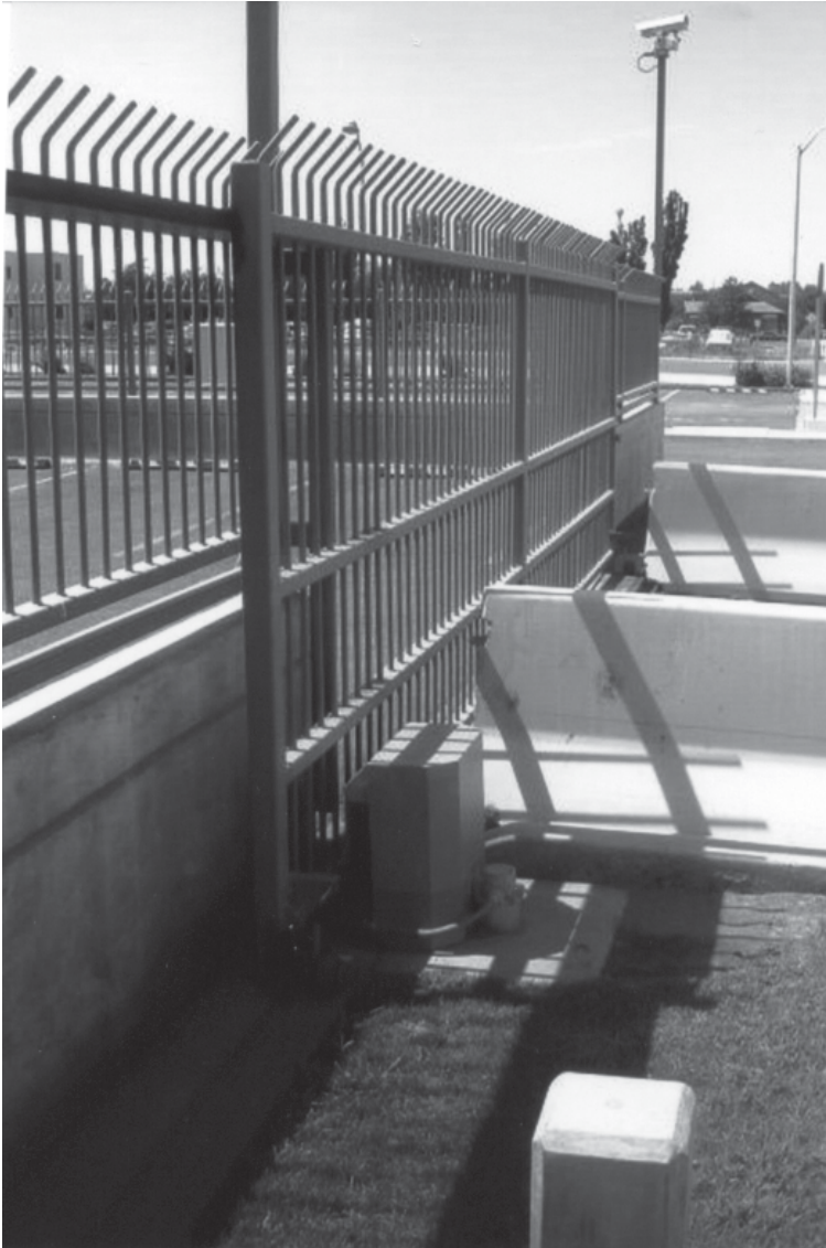
Figure 3-10. A sliding gate is an efficient barricade. This photograph shows the gate chain operator for a sliding wrought iron gate. Note that jersey barriers have been placed to force a vehicle to approach the gate directly. (Photo by Robert Reid, 2004)
