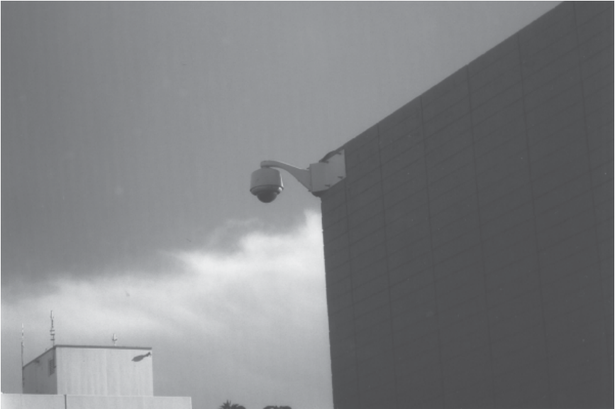
Figure 11-2. Outdoor dome camera. (Photo by Robert Reid, 2004).
