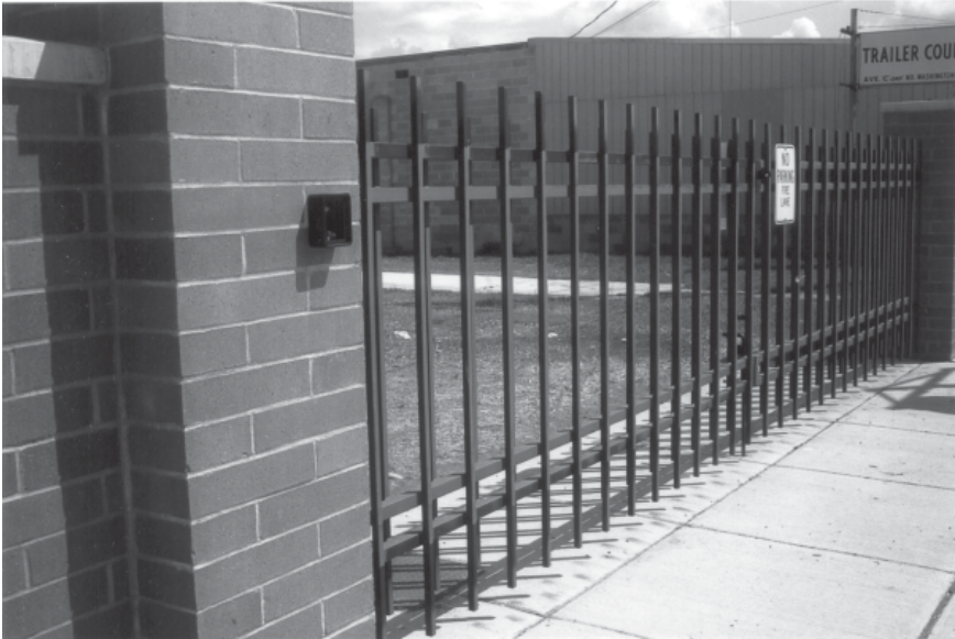
Figure 3-7. Typical wrought iron fence. (Photo by Robert Reid, 2004)
