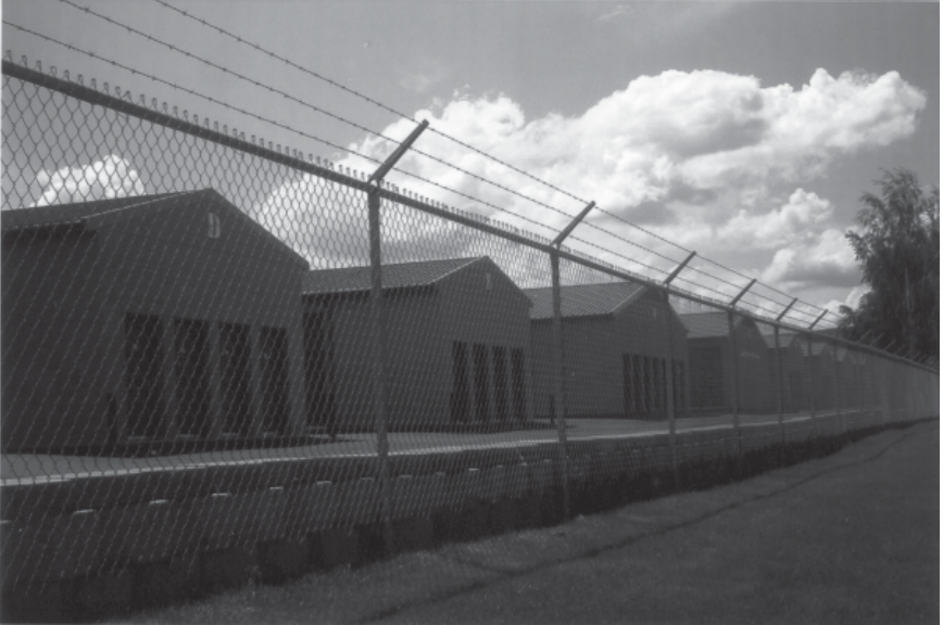
Figure 3-4. Chain link fence is an effective barrier for marking a boundary. This figure shows a typical 5-foot-high chain link fence being used for a commercial storage facility. (Photo by Robert Reid, 2004)
