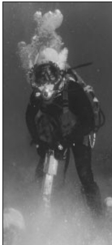
Figure 6-4. Underwater Construction Diving.
