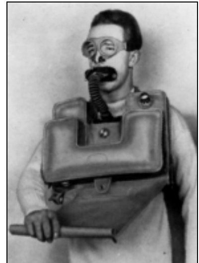
Figure 1-10. Original Davis Submerged Escape Apparatus.
