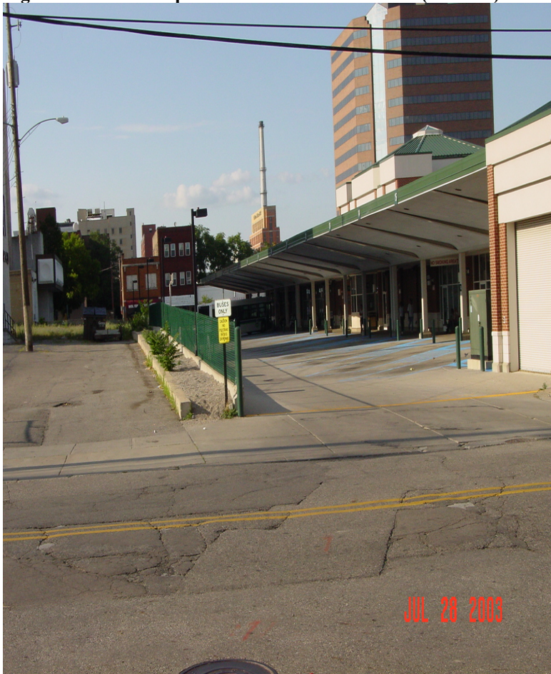
Figure 10.4. #1 Hot Spot Exterior of Bus Terminal. (Photo C)
