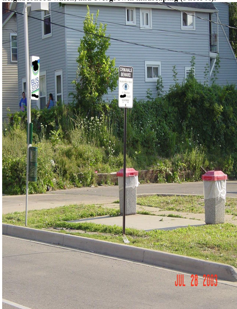
Figure 10.5. #2 Hot Spot noting multiple trash receptacles, neighborhood watch, and overgrowth landscaping (Photo A).
