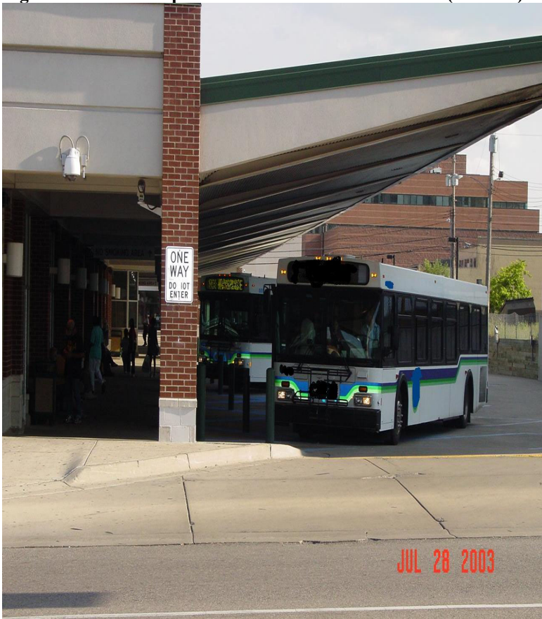
Figure 10.3. #1 Hot Spot exterior of main bus terminal. (Photo B)
