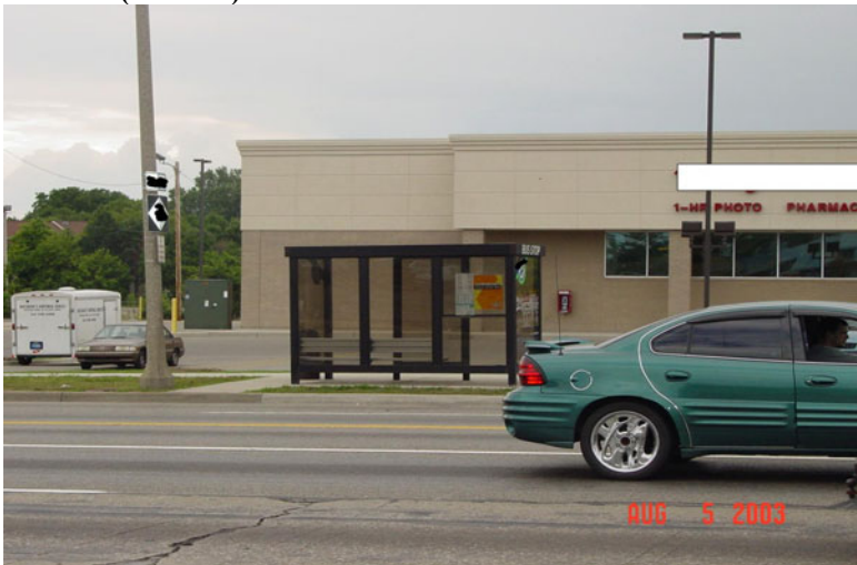
Figure 10.14. #5 Hot Spot noting a second bus stop shelter location. (Photo B)
