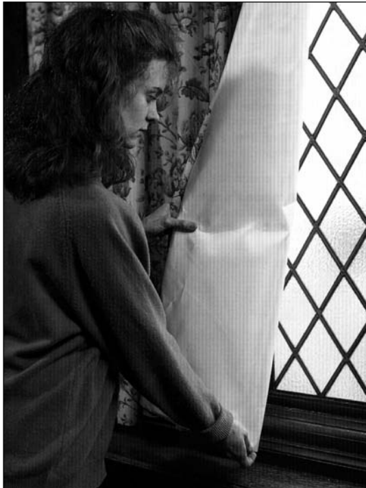
Above - bomb suppression lining for curtains. A cheaper alternative to some more expensive options and aesthetically more pleasing than coating the windows with film.
