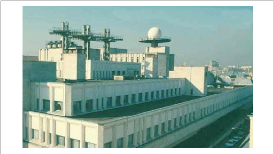
Figure 15-3. Special Communications and Information Service Moscow headquarters ( http://fso.gov.ru )
