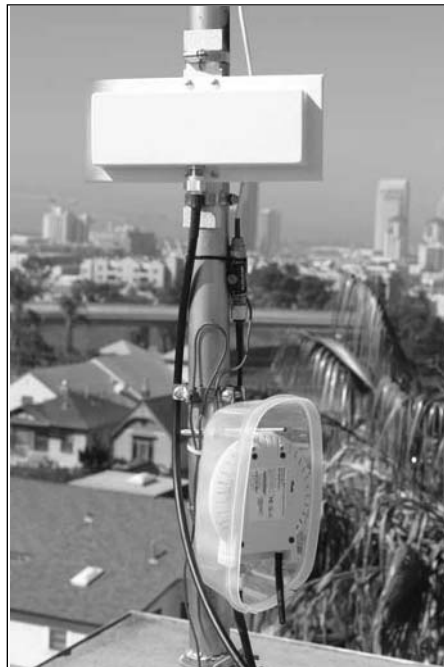
Figure 4.22 8571 with the Lid Removed
