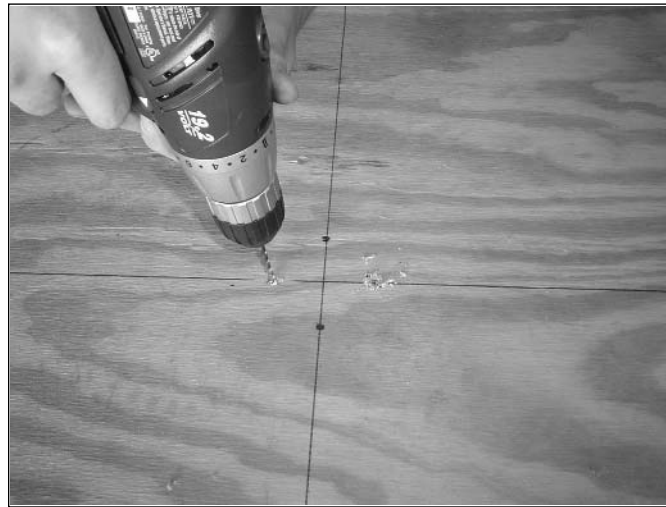
Figure 11.12 Drilling Pilot Holes for Lag Bolts
