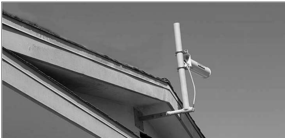
Figure 11.15 An Inexpensive Wall Mount Antenna Mast Made From Scrap Steel
