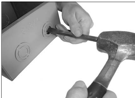
Figure 11.7 Using a Punch and Hammer to Remove Knockouts
