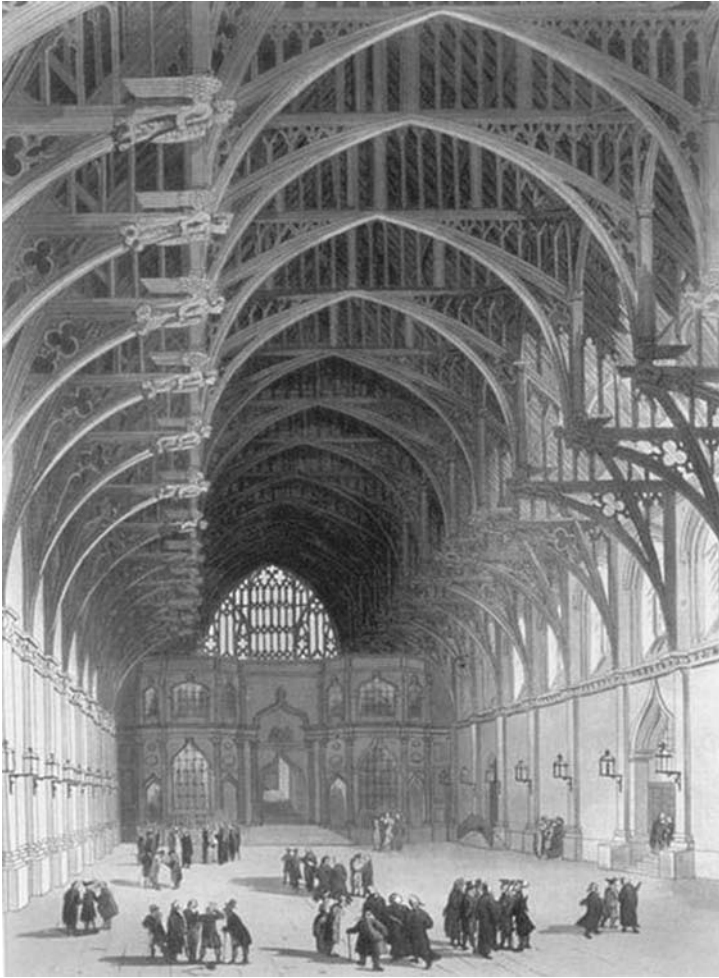
Figure 2.5. Westminster Hall, hammer-beam roof structure (c.1399).
