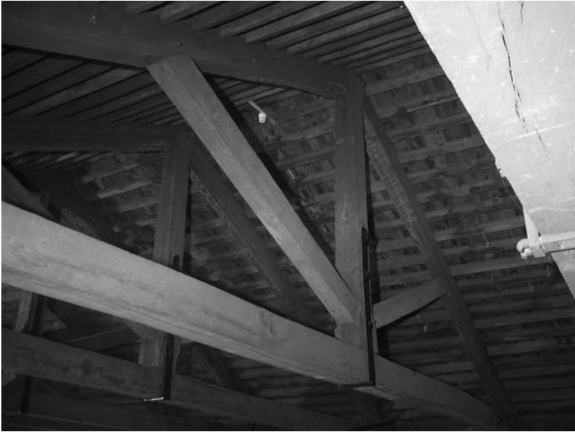
Figure 2.3. St Paul's Cathedral, roof truss over the nave.
