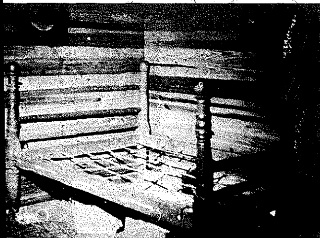
PLATE 201 A rope or "corded" bed in Aunt Arie's house. A shuck mattress fits on top of the ropes, which are woven through holes drilled in the frame of the bed.
