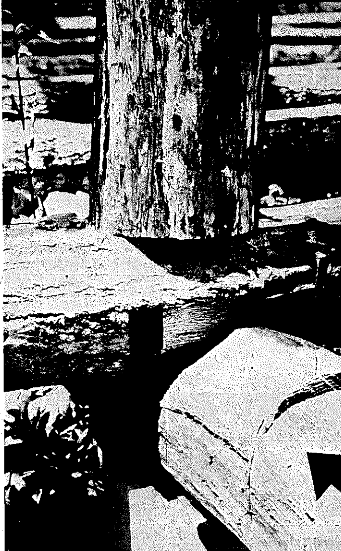
PLATE 50 This middle sill (arrow) is supported by two rocks.
