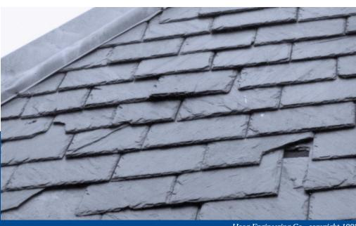
Slate roof damaged by hail.
