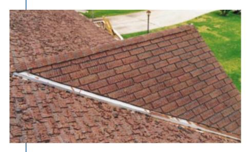
Asphalt roof shingles damaged by hail.
