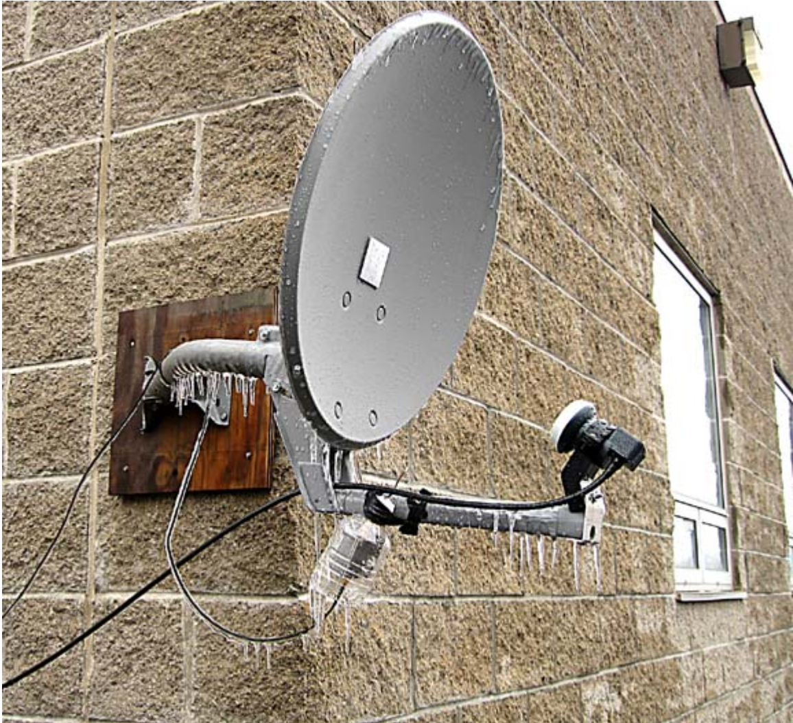
Figure 2. When correctly assembled the LNBF should be 13" ( \pm 0.25 ") from a point 9" up from the bottom edge of the reflector. The LNBF should point towards a point 9" from the bottom of the reflector rather than right at the center. The bottom edge of the front LNBF should be 10" ( \pm 0.25 ") from the bottom of the reflector.
