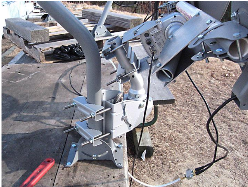
Figure 23 Example mount configuration. Note the use of a sturdy base tie point.
