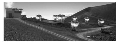
**Fig. 9.9** The Sub Millimeter Array (SMA) consists of eight 6-m antennas that are designed to operate to 0.3 mm, with a total geometric collecting area is 226 m<sup>2</sup>. The SMA is located on Mauna Kea, at an altitude of 4.1 km. It was built and is operated by the Harvard-Smithsonian Center for Astrophysics (CfA) and the Academia Sinica Institute for Astronomy & Astrophysics (ASIAA), Taiwan (photo courtesy of N. Patel, CfA.)
