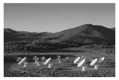
**Fig. 9.8** The Combined Array for Research in Millimeter-wave Astronomy (CARMA) is located in northern California, at an elevation of 2.2 km. CARMA is the merger of the Owens Valley Radio Observatory (OVRO) millimeter array (consisting of six 10-m dishes) and the Berkeley-Illnois-Maryland Association (BIMA) array (consisting of nine 6-m dishes). Funding for CARMA is provided by the U. S. National Science Foundation and the consortium universities (photo courtesy of J. Miller and D. Bock)
