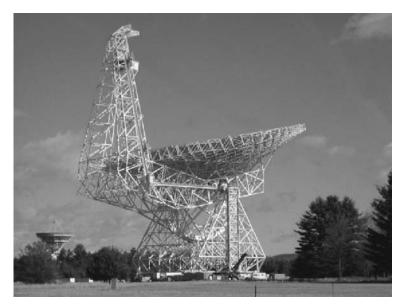
**Fig. 7.11** The Green Bank Telescope (GBT) at West Virginia, U.S.A. The telescope is an off-axis paraboloid with a 110 m by 100 m diameter. This design was chosen in order to minimize side lobes and reflections in the telescope structure that lead to instrumental artefacts or "baseline ripples"
