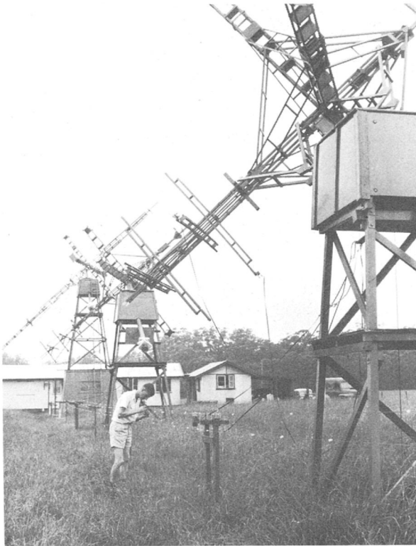
Fig. 13 J. P. Wild adjusting the transmission line of one of the three dual-polarization rhombic antennas of the Dapto spectrometer (1952).
