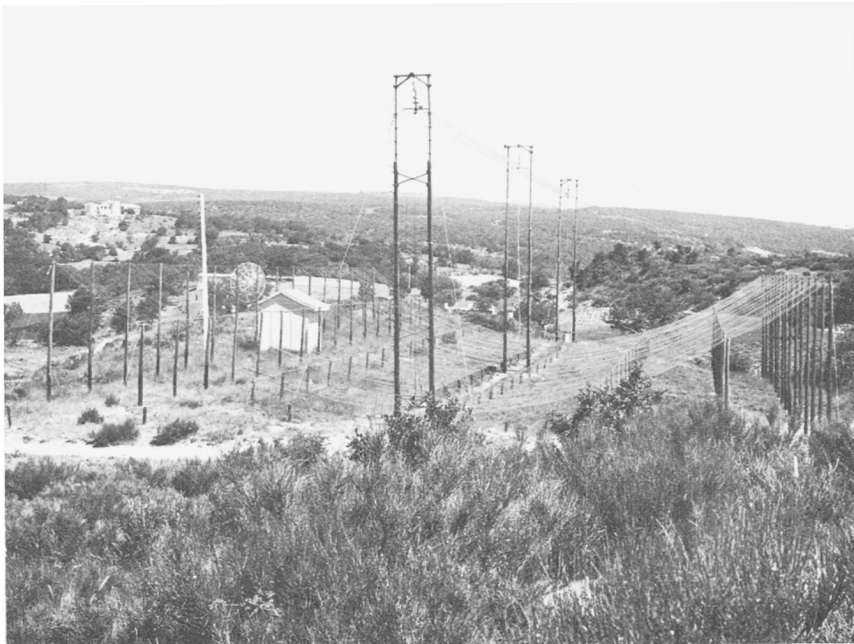
Fig. 7. One antenna of the Saint-Michel Interferometer of the Paris Institute of Astrophysics (CNRS) was used at 300 MHz for survey of radio sources (1959).
