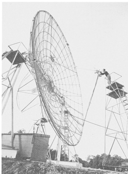
Figure 3 36-ft paraboloid at Potts Hill, near Sydney, c. 1953. The telescope is mounted as a transit instrument. Brian Robinson is seen working on the receiver.
