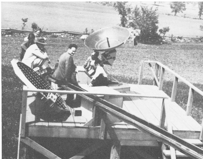
Figure 2. Inspection of the 10.7 cm solar patrol radio telescope at the Goth Hill Radio Observatory during an AAS meeting held in Ottawa, June 1949. The radio black box and quarter-wave plate may be seen at the front of the platform. Counterclockwise: W.J. Medd (under reflector), C.L. Seeger, A.H. Shapley, J.F. Denisse, J.P. Hagen and A.E. Covington. (Photo courtesy Grote Reber)
