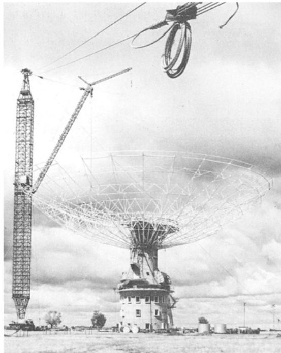
Fig.10 The Parkes 64 m telescope in course of construction, 1959.
