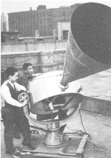
Fig. 2. First experiment to receive solar noise, at 3300 MHz, by M. Oda (front) and T. Takakura (back) at Osaka University in November, 1949.
