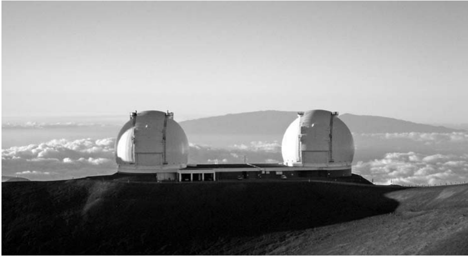
Figure 3.2. The twin domes of the W.M. Keck Observatory on the summit of Mauna Kea. Each dome encloses a telescope with a segmented mirror having an effective aperture of about 10 meters. The domes are 85 m apart. Photo credit: author.
