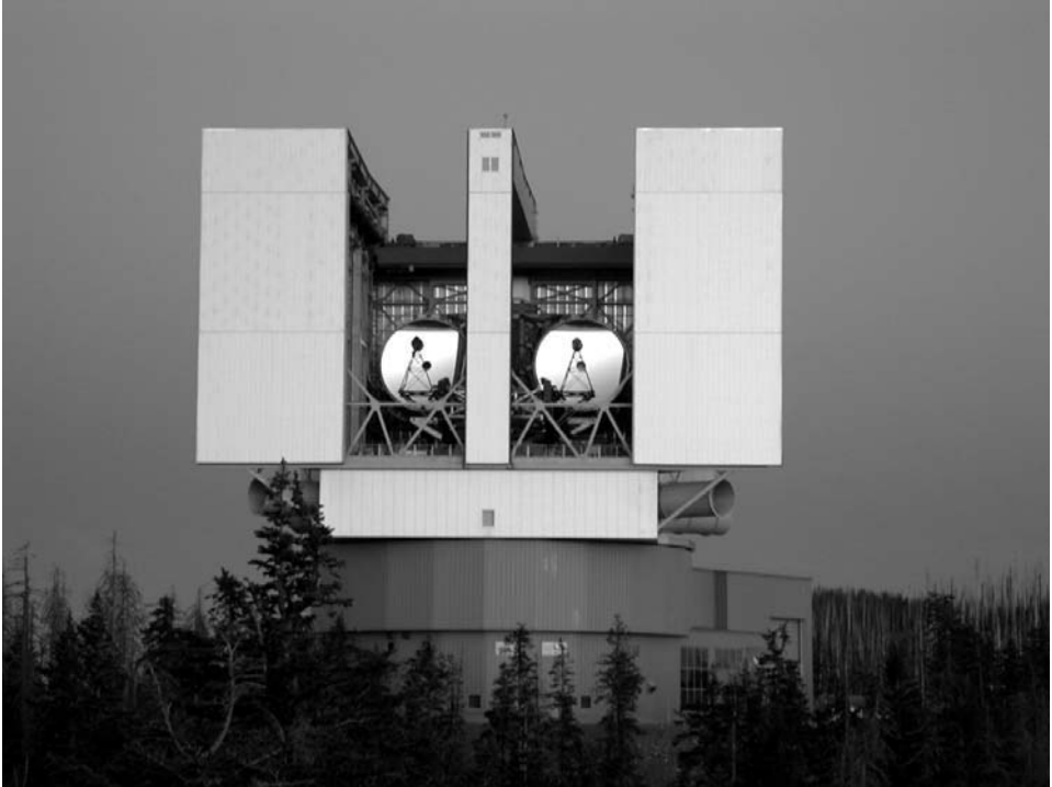
Figure 3.15. The Large Binocular Telescope on Mt. Graham with its pair of 8.4 m spin-cast primary mirrors installed. Credit: University of Arizona.
