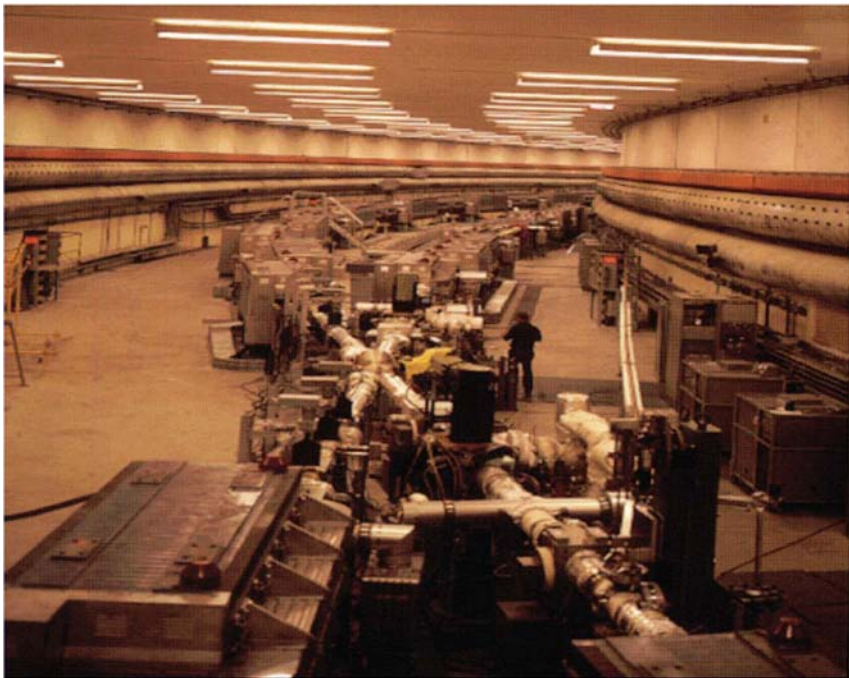
Fig. 7.27 View of the ISR at intersection point 5. (Courtesy of CERN).
