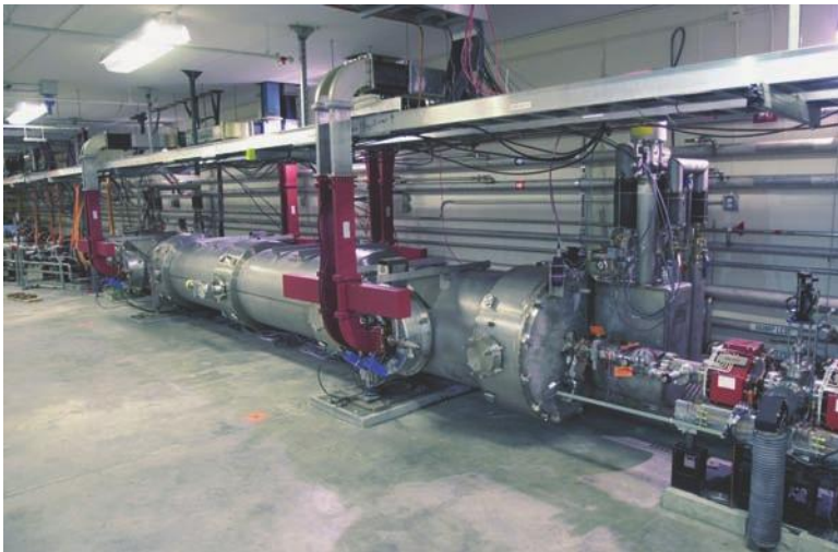
FIGURE 4.4 Niobium cavities inside a cryomodule with the RF waveguide feeds in red. The electron beam enters from the pipe in the right foreground.
