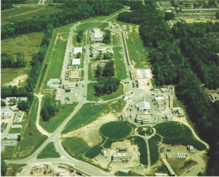
FIGURE 4.5 An aerial view of the Continuous Electron Beam Accelerator at Jefferson Lab. The FEL facility building is top center and CEBA is below ground in a 7/8 mile circumference oval. The nuclear physics end stations are in the three grass-covered domes at lower right. The cryogenic helium refrigerator is housed in the building group at the center of the oval.
