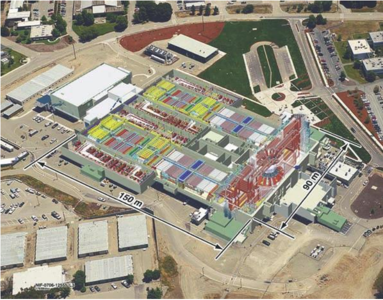
FIGURE 14.1 The National Ignition Facility (NIF) is approximately 150 m \times 90 m and seven stories tall. The roof has been “removed” from this aerial photo to show an engineering rendering of the laser. The two laser bays are shown on the upper left. The switchyard (in red) is shown on the lower right, as is the spherical target chamber (in silver) into which the 192 beamlines converge.
