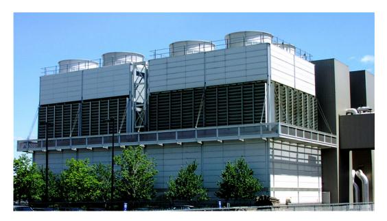
**Figure 11.2** A mechanical-draft cooling tower. The fans are located within the cylindrical housings at the top. Air is drawn in through the louvres on the side.
