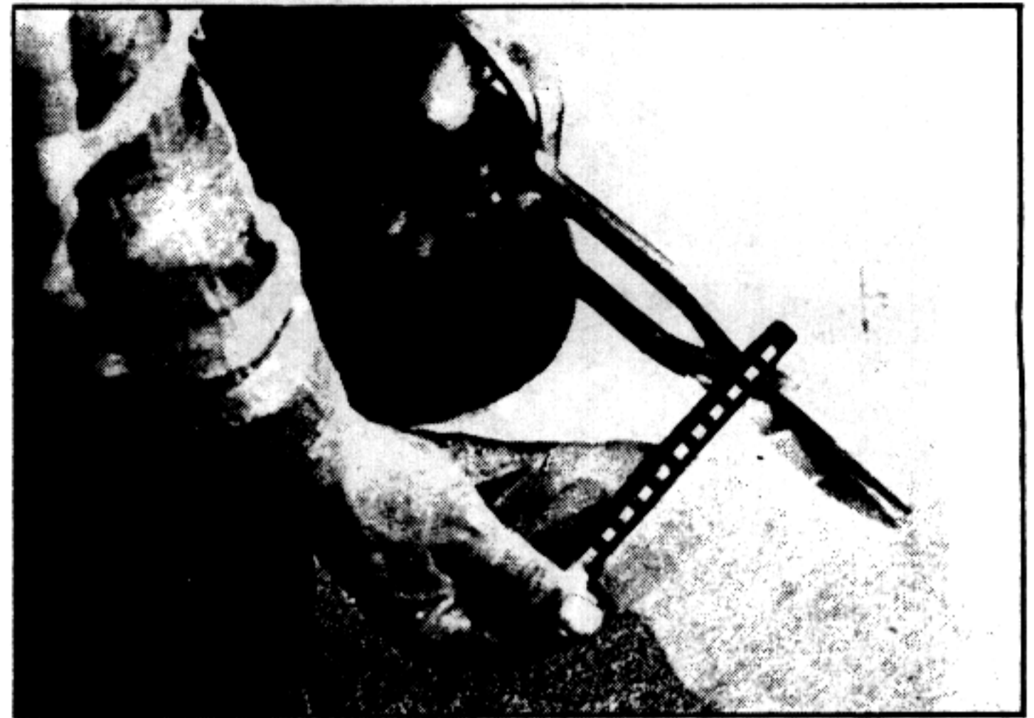
Metal screen is cut to proper width, using sleeve as guide.
