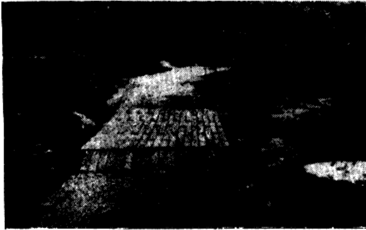
Figure 7.--Note the row of rocks on top of bridge beam at the foot of the bridge. This is typical of the warning signs used by the VC/NVA to warn of their mining activities.
