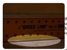
If your existing floor is uneven, use a straight edge to locate the low spots, which will create a gap underneath the straight edge.
