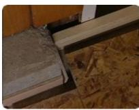
A jigsaw makes cutting out the notch quick and simple.
