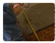
When you come to the end of your first row, you will probably need a piece smaller than a full panel to fill the remaining space. Simply measure the space, set your table saw fence to the required dimension, and then make the cut. A hand held circular saw or jigsaw can also be used to make these simple cuts.
