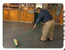
Remove any bubbles or ripples with a push broom, working from the center to the edges. This new flooring is tough, durable and good looking. If you ever plan to park a car on this surface, it is resistant to oil and gasoline.
