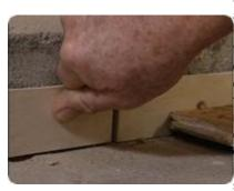
This is called a floating floor system, which means it is not attached to the concrete underneath, but instead sits or floats on top. This entire floor expands and contract with changes in humidity and temperature, which means you need to use spacers around the edges of the floor to create a quarter inch gap. When the floor installation is complete, the spacers can be removed so that the gap enables the floor to move as it needs to.
