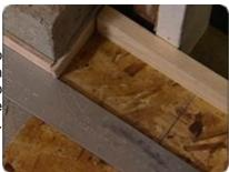
The easiest way to do this is to set the panel in place and then use a straight edge or square to extend the wall lines onto the board.
