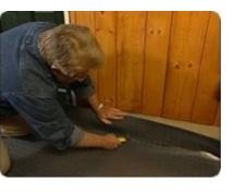
Carefully remove the protective liner from only one side, because you want the tape to stick only to the covering and not to the underlayment. This leaves the floor covering free to expand and contract with changes in temperature and humidity.
