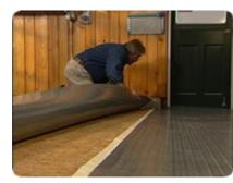
Because Ron was installing his floor in a garage and workshop he decided on something called the G-floor from Better Life Technologies for his floor surface. This garage floor covering comes in nine-foot widths and simply rolls out, but it lies perfectly flat and stays in place without the need for adhesive.
