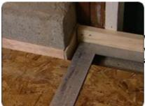
When working in a doorway, you will need to notch out a panel to fit around the corner.
