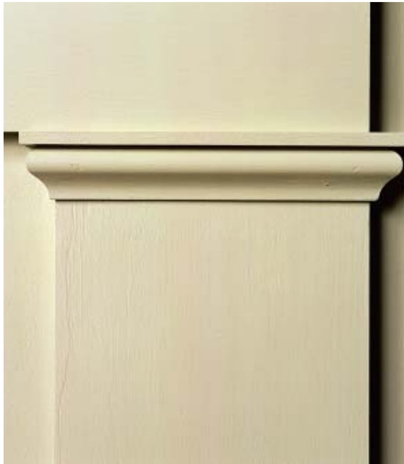
This detail shows the capital molding that caps the pilasters.
