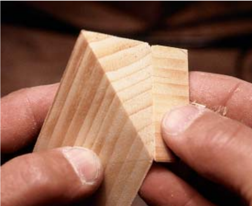
A small block is glued to the angled cove blocking. This supports the cornice molding return piece.
