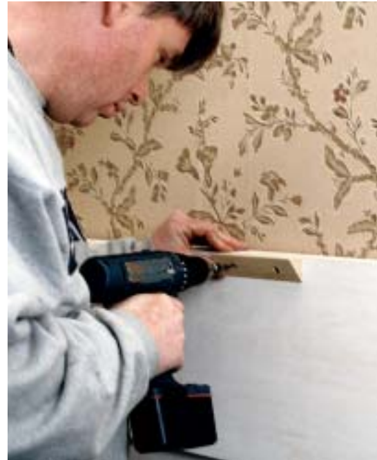
Screw angled cornice blocks along the top edge of the architrave.
