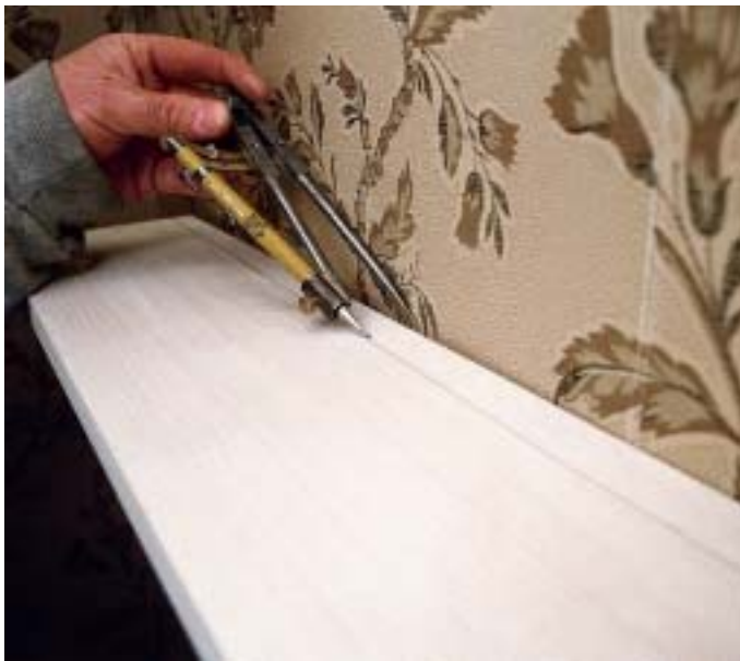
After setting the legs of the compass to the widest gap between the mantel shelf and the wall, drag the compass along the length of the shelf. Here the mantel shelf is still oversize, so the scribed amount is a full inch larger than the widest gap.
