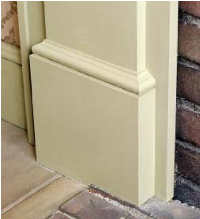
This detail shows the plinth with the torus molding.
