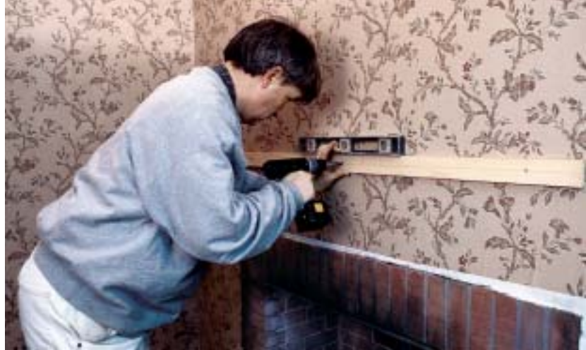
Furring strips, shimmed plumb as needed and attached to the wall surface, provide good solid support for the foundation. Use the appropriate fastener based on the wall material.
