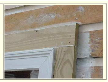
Note how there is primer behind the casing. Prior to installing these boards I scraped off the old paint in the scalloped grooves, sanded the wood clean, and applied primer. This is just a precaution in case water gets behind the trim someday. Primed wood is less able to absorb water.
