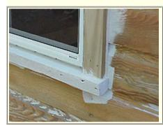
The bottom end of the side casings were cut at a 10 degree angle to match the window sill.
