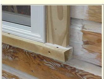
I installed 1x4 treated pine on the sides. The lower edge of this piece was cut at the same 10 degree angle, so it mated with the sloped sill.
