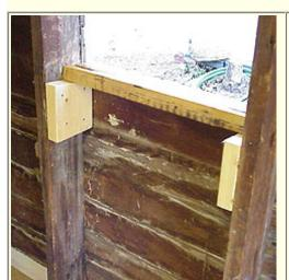
After the sill was stripped and sanded, I installed two angled blocks for the sill to rest on. I was careful to make sure that the sill would end up level, because the window will rest on this sill.
