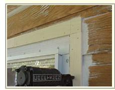
Using a brad nailer, I attached some 1/4" thick strips of wood around the perimeter of the window.
