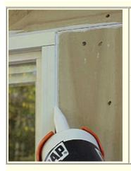
I applied caulking all over the place, especially between the window frame and the wood casing.
