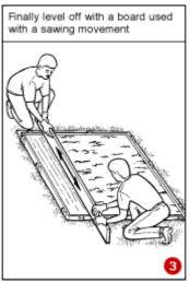
If rain is expected cover the concrete with polythene for 24 hours. In warm weather cover it with wet sacks and sprinkle them with water over the 24 hour period. The base is then ready for the shed.
