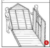
Have a helper raise the panels into Check each panel to ensure you will be fixing them in their correct positions - doors and windows in the right place (5).
