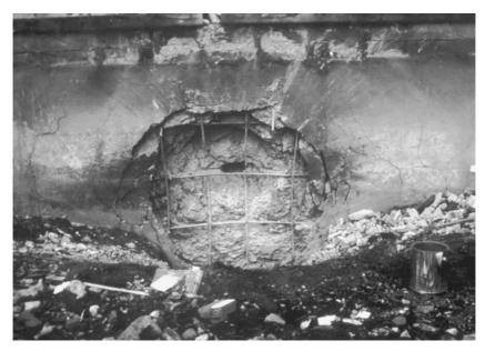
**Figure 10.5** Seat of an explosion. The cratering effect created by a blast is called the seat of the explosion. In this instance, this seat was created by a high-order detonation placed against a building foundation.
