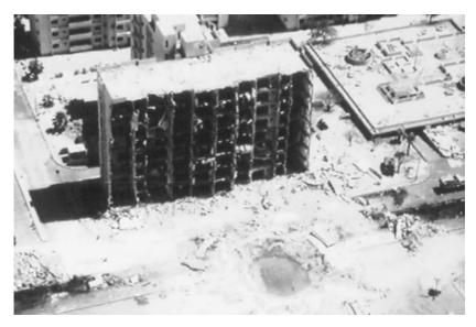
**Figure 10.3** The water-filled bomb crater in front of the troop barracks, Khobare Towers. The building was virtually destroyed by a large vehicle-borne IED. (Courtesy of F. Guerra.)
