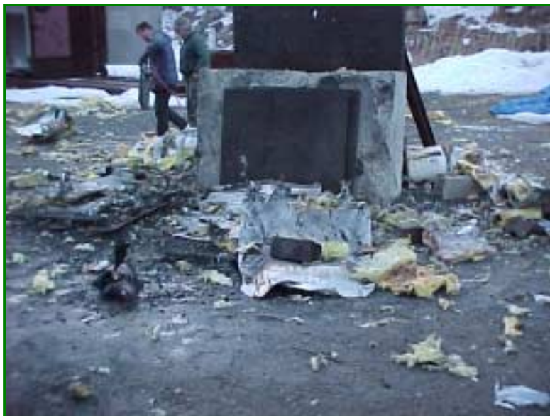
Figure 31 – Comp A5 Post Test
