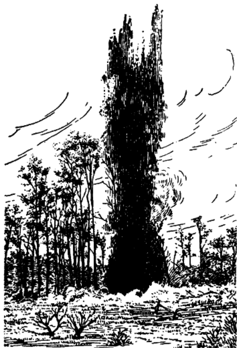
Fig. 143.—A short test shot for ditch blasting. Note how the excavated ground is lifted and scattered.
