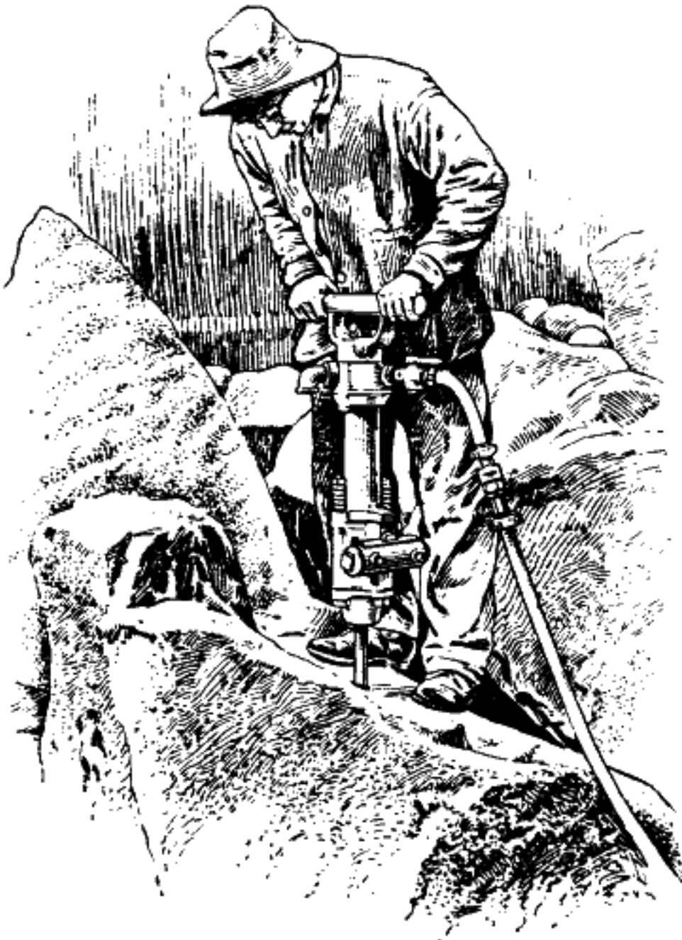
Fig. 72.—Hammer drill on road work.
