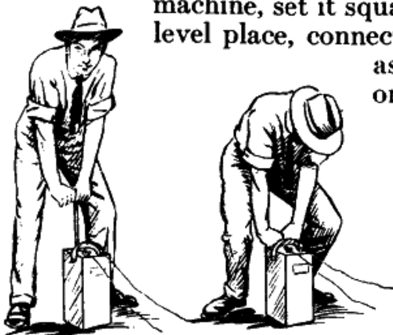
Fig. 60.—Operating a push-down Blasting Machine.
