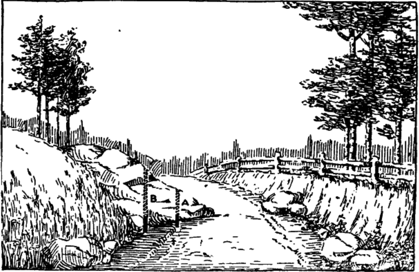
Fig. 97.—Blasting out a high side, "A" should be fired before "B." Where the high side continues along the road for some distance each set of holes should be fired together by the electric method.
