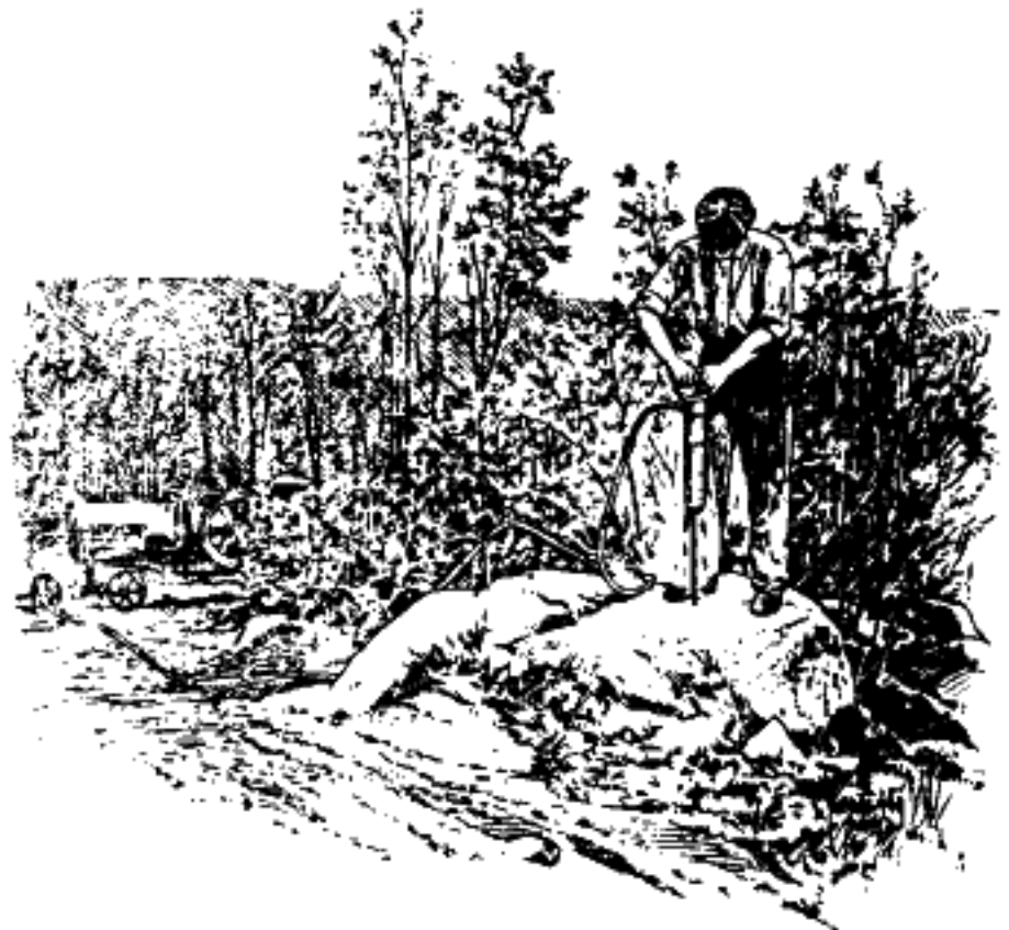
Fig. 77.—Portable compressor supplying air to hammer drill.
