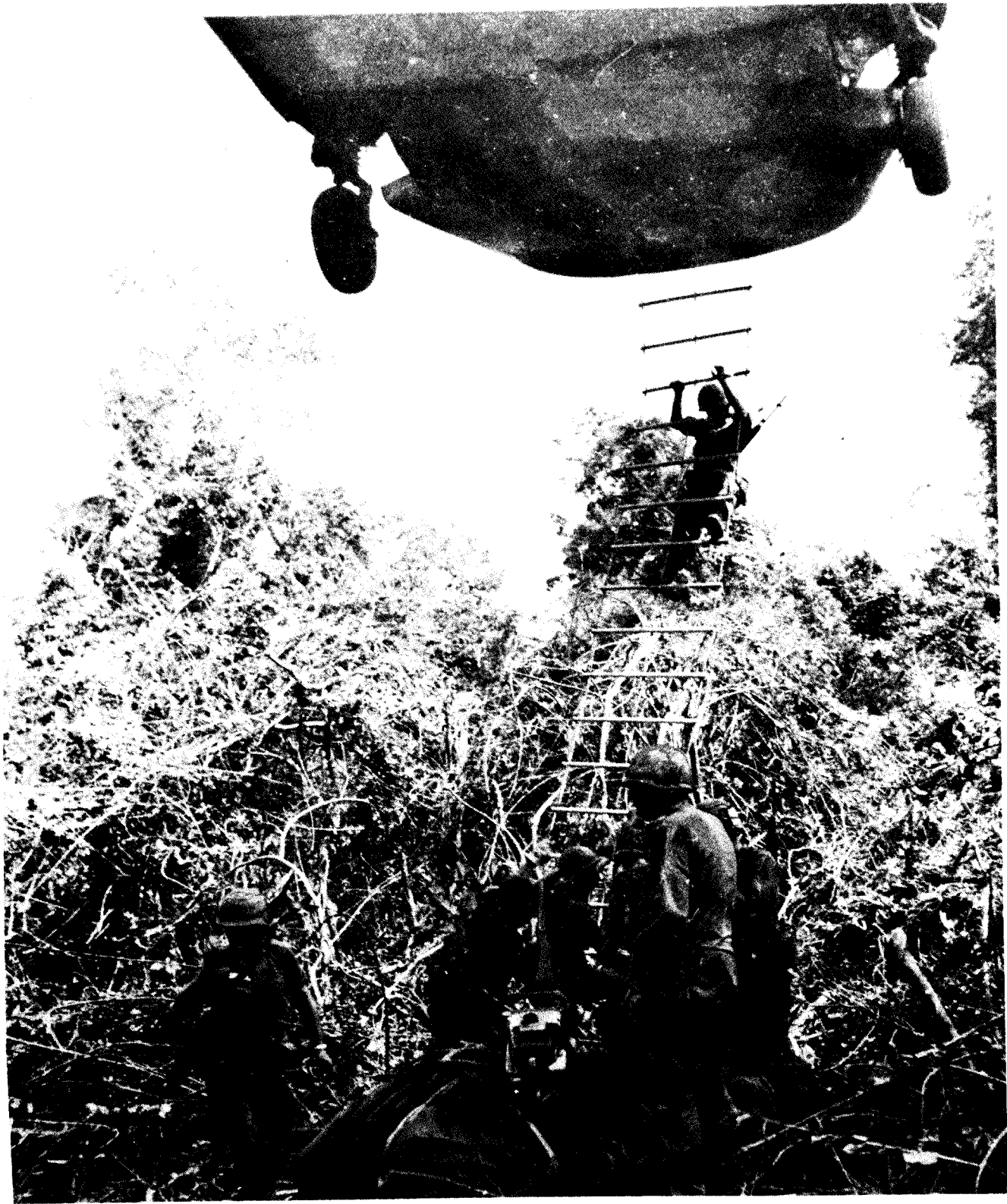
Figure 4-1. Combat engineer landing zone clearing team descending from a hovering Chinook (CH47).
