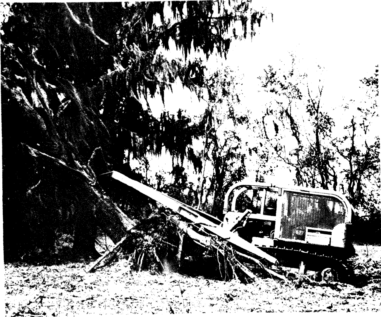
Figure 3-6. Medium sized tree being felled with a knockdown beam-bulldozer blade combination.
