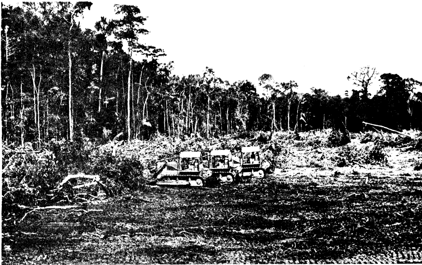
Figure 3-33. Multiple tractor piling operation using angled cutting blades.
