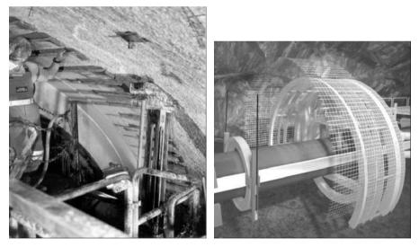
Fig. 4.13. left: Anchoring behind the cutterhead; right: Installation of wire mesh behind the cutterhead  $^{10}$
