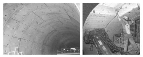
Fig. 4.32. Segmental tunnel lining<sup>30</sup>; Placing of small discs of wood in the joint
