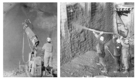
Fig. 5.3. Spraying concrete – wet mix mode
