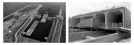
Fig. 10.2. Pre-fabricated tunnel blocks for Øresund tunnel<sup>4</sup>
