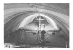
Fig. 2.6. Supply and extract channels above the carriageway. The separating vertical wall has not yet been mounted.<sup>14</sup>
