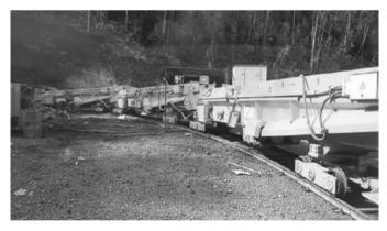
Fig. 4.68. Mucking with continuous conveyor<sup>63</sup>
