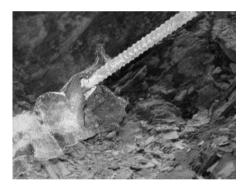
Fig. 5.14. Anchor rod within geotextile containment
