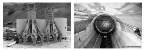
Fig. 11.5. Shaft Sedrun, excavation gripper; view into the lined  $shaft^6$
