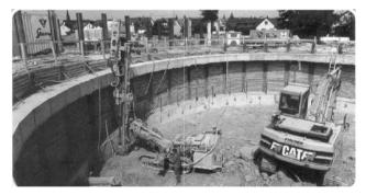
Fig. 11.6. Launch shaft, city rail extension Stuttgart airport
