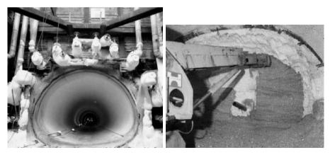
Fig. 6.9. Soil freezing: main collector Mitte Düsseldorf, Germany
