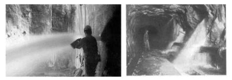
Fig. 8.2. Water inrush. Left: Füssen tunnel<sup>12</sup>; right: Simplon tunnel<sup>13</sup>
