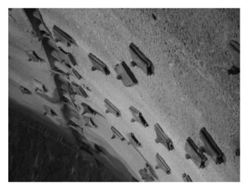
Fig. 14.29. Anchor headplates and pipe array
