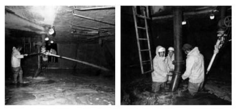
Fig. 10.4. Work chamber of a pneumatic caisson (Metro Amsterdam)
