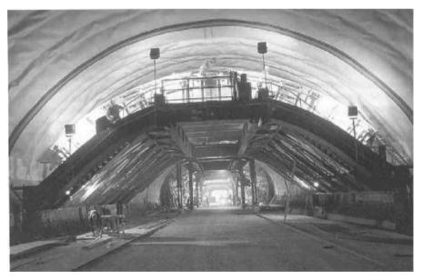
Fig. 5.30. Rolling formwork (Engelberg base tunnel)<sup>26</sup>
