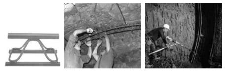
Fig. 5.23. Lattice girder (Pantex-3-arch), connecting the segments, mounting with rock bolts
