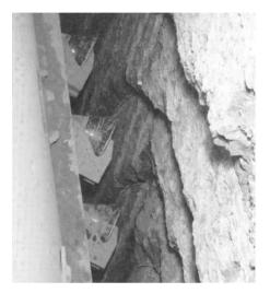
Fig. 4.63. Undercutting at the Uetliberg tunnel<sup>58</sup>
