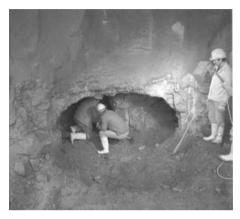
Fig. 8.1. Karst cavity encountered at the excavation of the Rollenberg tunnel<sup>3</sup>
