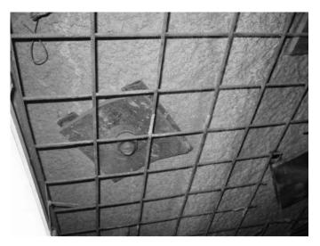
Fig. 14.30. Squeezed anchor headplate. The two steel tubes had initially circular cross sections. Their squeezing indicates that this anchor has been overloaded.
