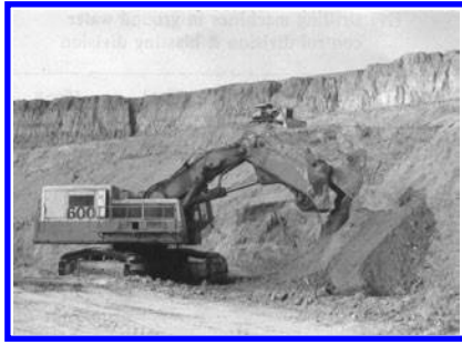
Figure 6.7 A hydraulic excavator working at Civil site.
