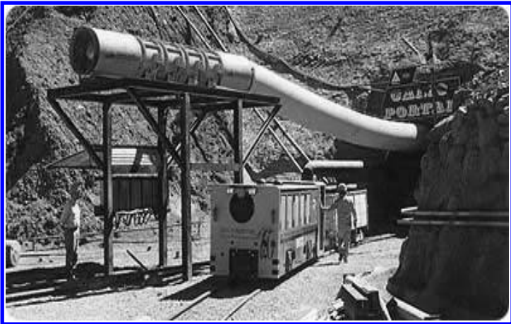
(f) Diesel locomotive with ventilation arrangement at the portal of a tunnel – A track system layout. (Courtesy: GIA Industry)
