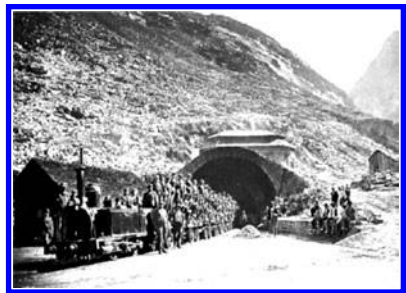
(f) A tunnel portal
