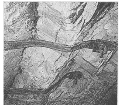
Straps, when used, should be placed across the 'grain' of the rock as shown
