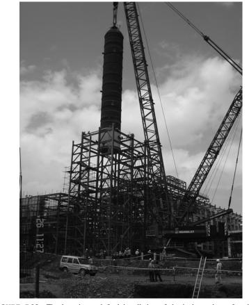
**FIGURE 7.23** The lowering and final installation of the hydrocracker referred to in Figure 7.22.
