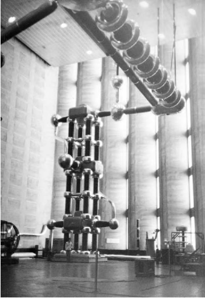
Figure 2.14 Testing transformer for 1200 kV r.m.s. comprising three single unit transformers according to Fig. 2.13, with metallic tanks and bushings (High Voltage Laboratory, Technical University of Munich, Germany). (Note. Suspended at ceiling and connected with transformer is a selenium-type rectifier with a reverse voltage of 3.4 MV, see ref. 5.)
