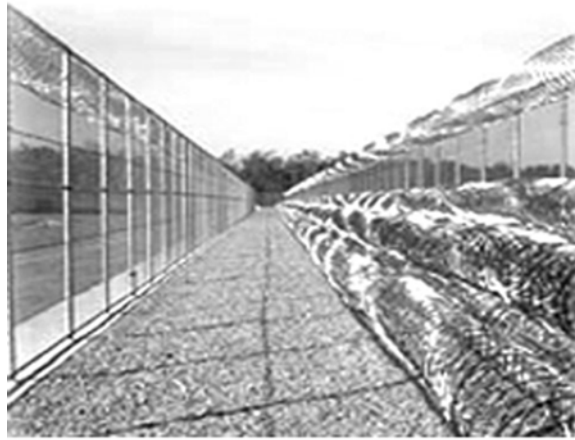
Prison Perimeter Fence: Double Layer With Razor Wire, Motion Sensors, High Voltage And Vibrating Machines To Destroy Tunnels
