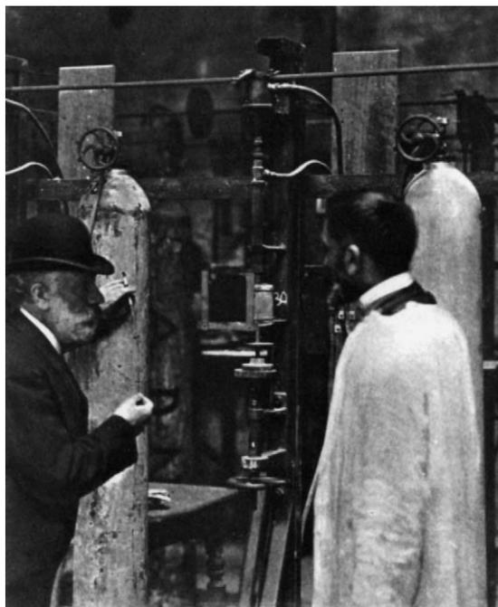
Fig. 10. Prof. Verneuil (left) and Mr. Spec-Torsky in front of a flame fusion apparatus about 1910 (from Ref. [2]).
