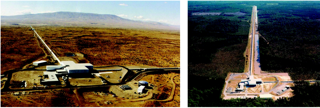
FIGURE 6.4.1 Aerial photographs of the interferometers used in the Laser Interferometer Gravitational Wave Observatory (LIGO). The long tunnels house the evacuated laser chambers, in which laser beams travel a 4-km path length. At the vertex of the L, and at the end of each of its arms, are test masses that hang from wires and that are outfitted with mirrors. Ultrastable laser beams traversing the vacuum pipes are used to detect the ultras-small change in the separation of a pair of test masses caused by the passage of a gravitational wave. Images courtesy of the LIGO Laboratory.
